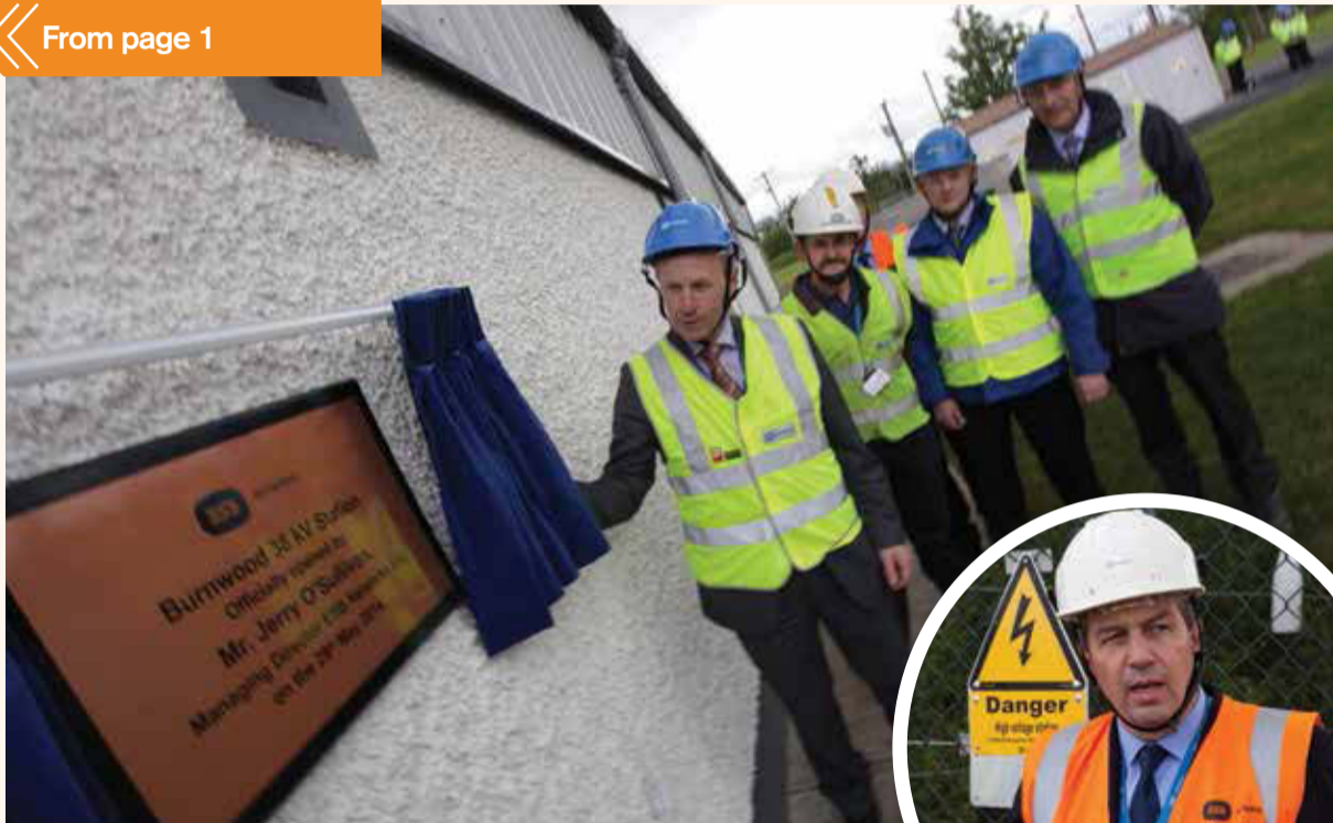
Jerry O'Sullivan, MD Networks, officially opens Burnwood 38 kV Station. Right: Alan Kelly, Training Operations Manager. Below right: Stephen McCarthy Operations Training Officer, explains the fault panel.
