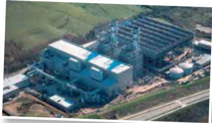
The Amorebieta plant in the Basque region of Spain.
