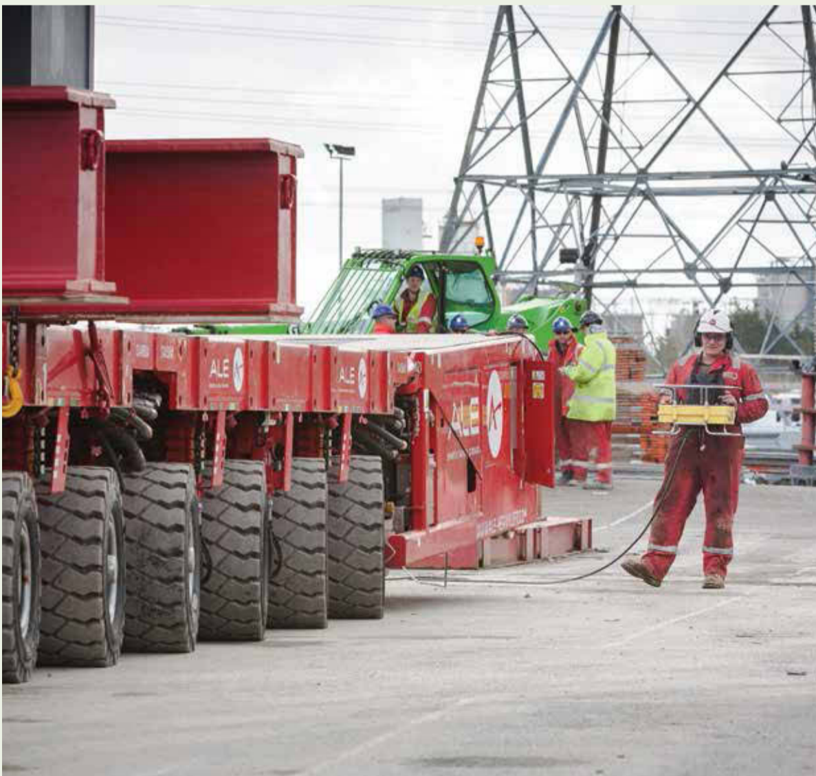
Moving the generator on the lorry via remote control is a delicate job. (All photographs by Greg Harding Photography).
