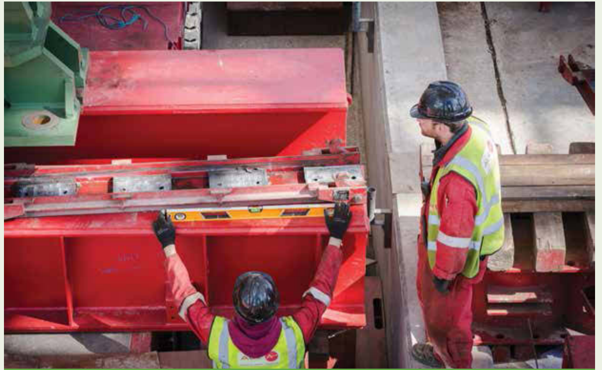
Checking everything is exactly level before starting to transfer the turbine and generator.
