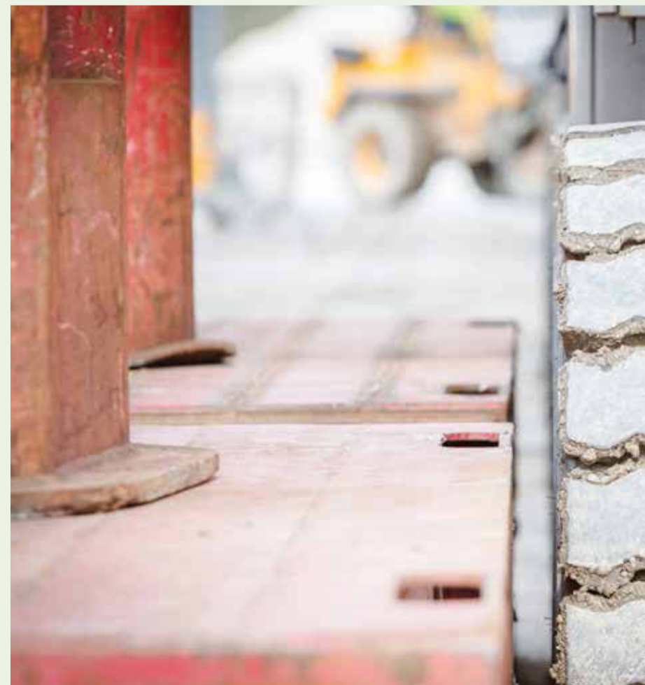
The lorry has to line up very precisely with the platform inside the turbine hall for the transfer to work.
