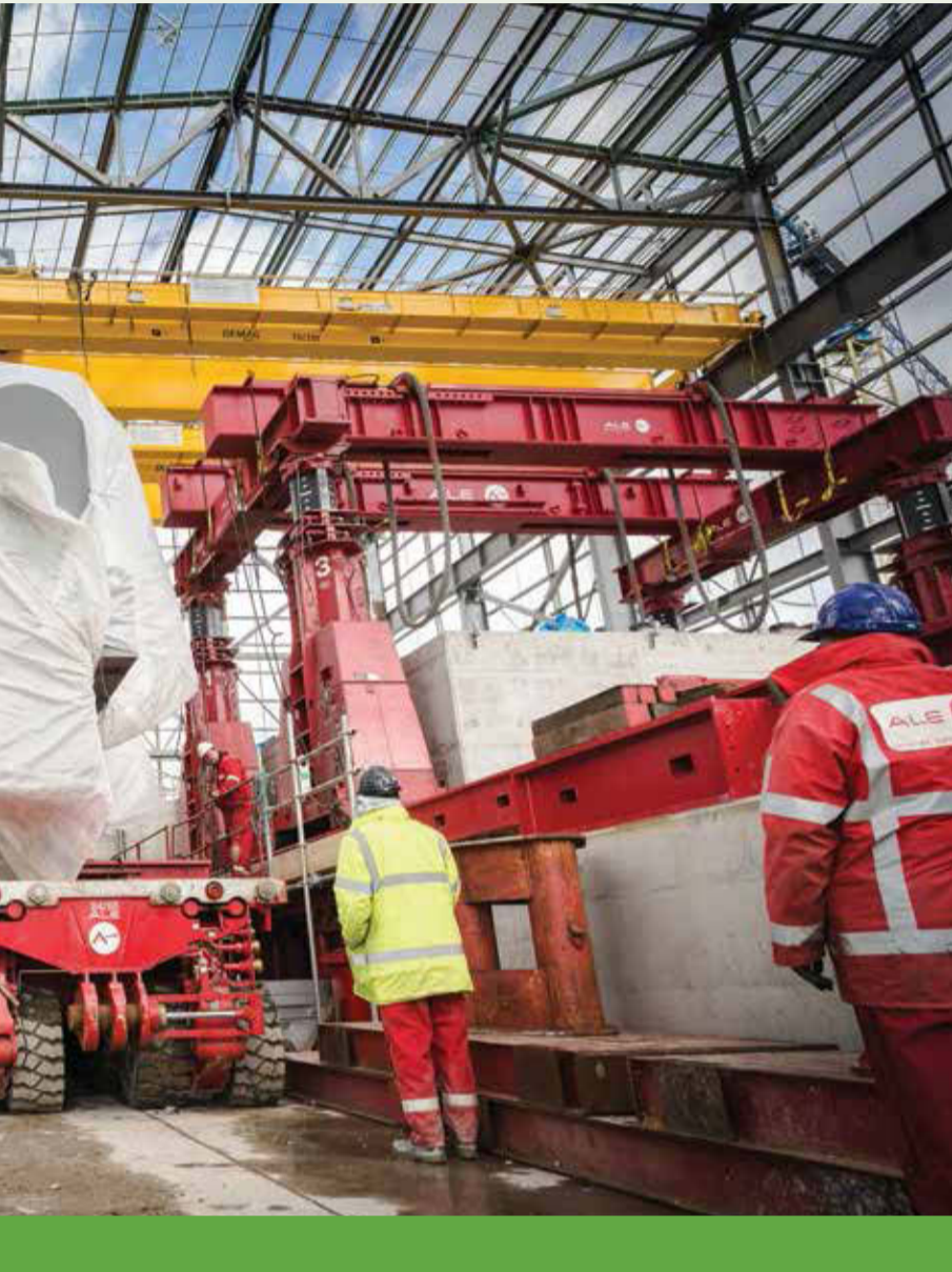
Checking everything is exactly level before starting to transfer the turbine and generator.
