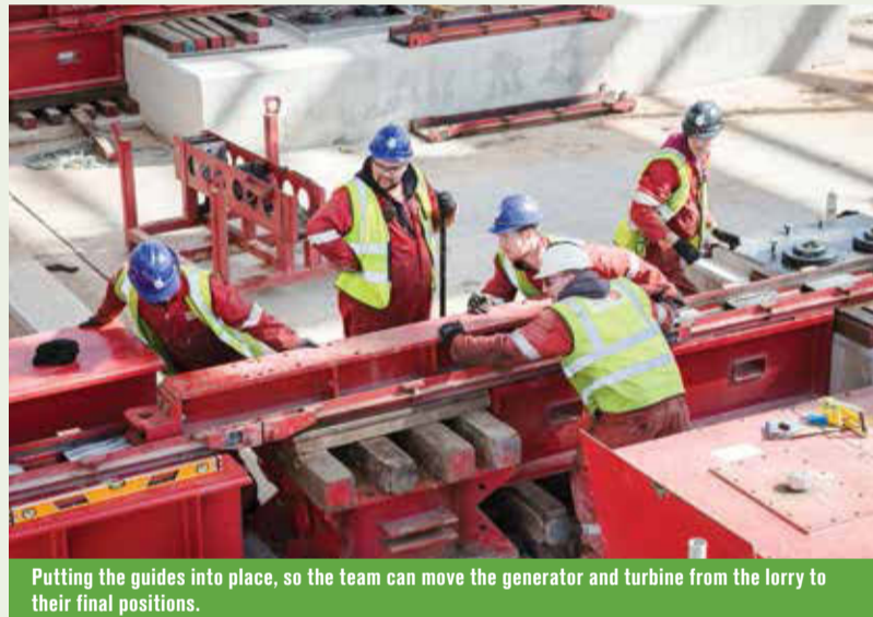
Checking everything is exactly level before starting to transfer the turbine and generator.
