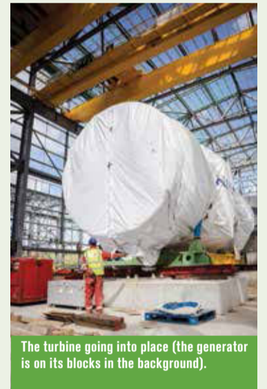
Putting the guides into place, so the team can move the generator and turbine from the lorry to their final positions.
