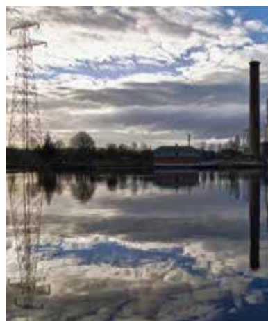
Marina Generating Station in Cork.
