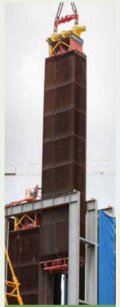
The heat exchange module is guided into the boiler housing.
