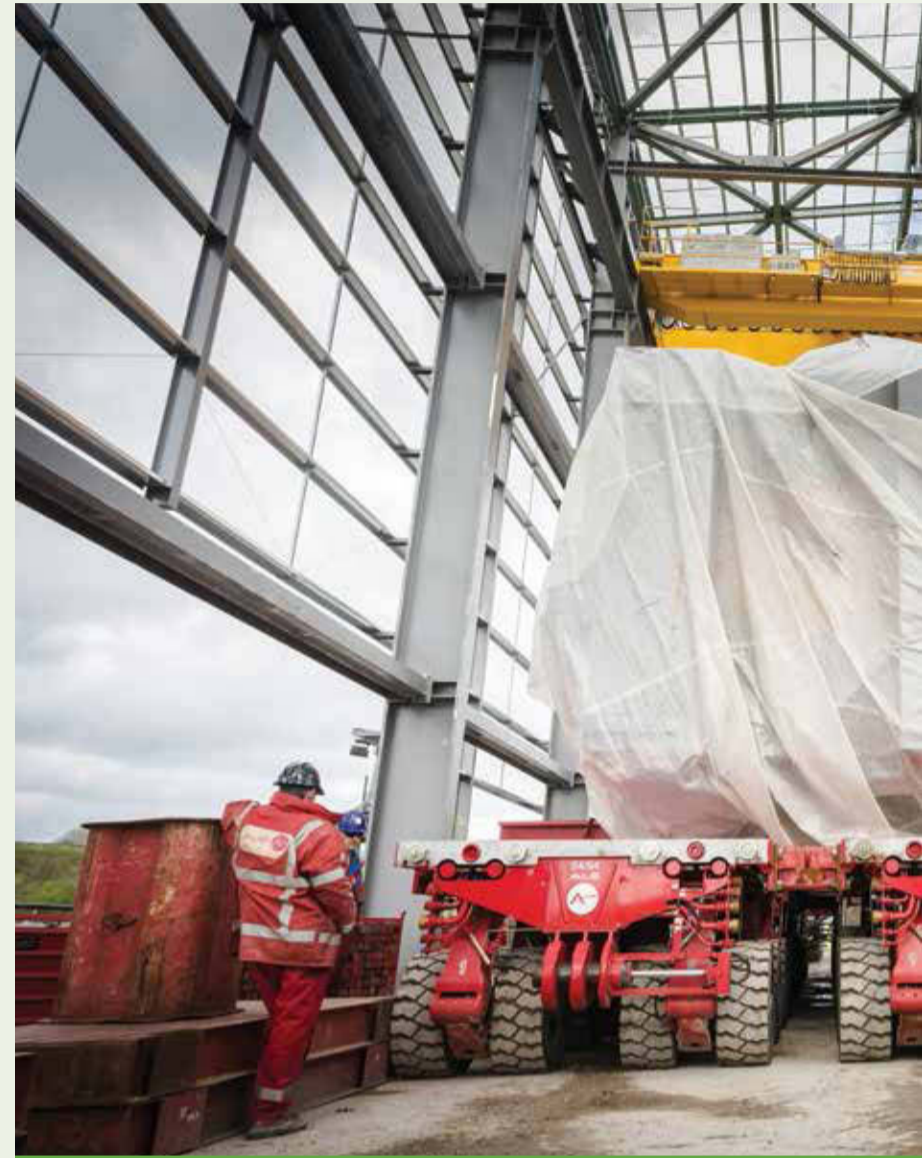
The generator enters the turbine hall.
