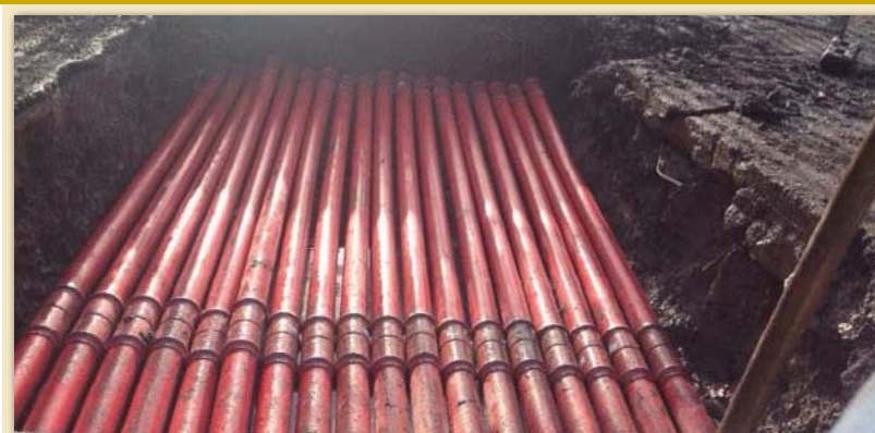
Crossing Centre Park Road at Marina entrance.
